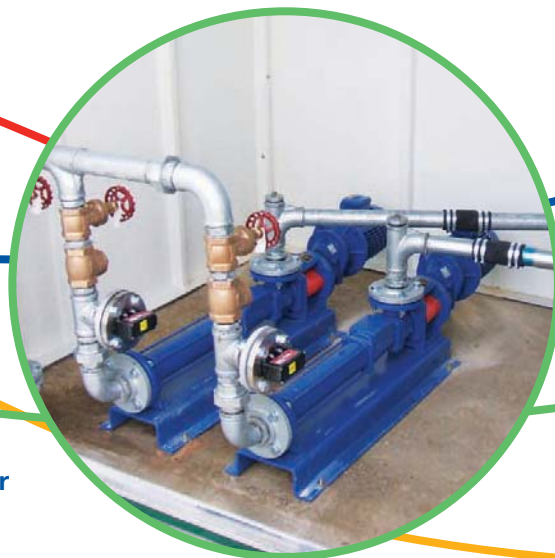
Waste water pumping
