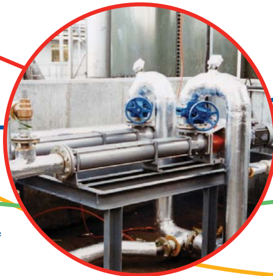
Pumping of slurry mix
